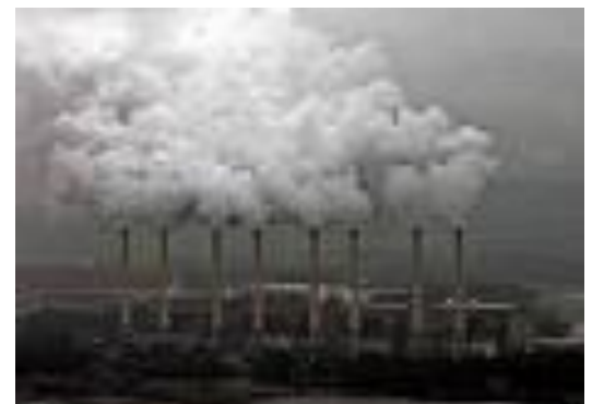
Hazelwood Power Station (Brown Coal)
